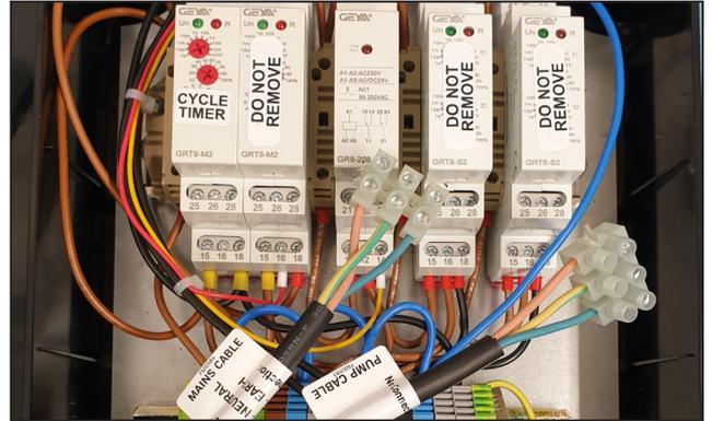
2. With the box front open, familiarise yourself with the connectors inside. The pump and mains cables are fitted with terminal blocks for easier connection to your pump and mains supply.
