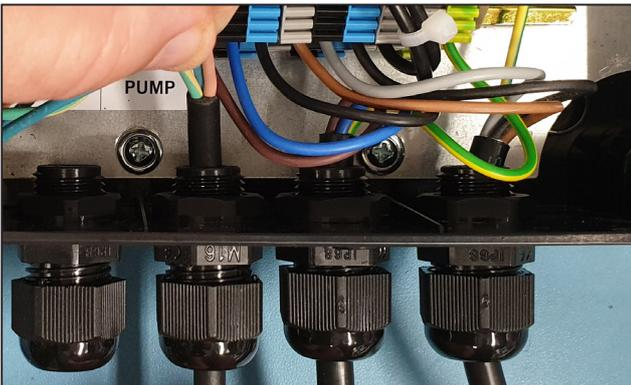
3. **PUMP CABLE:** Feed enough wire through the gland nut, into the control box to allow you to make the connections to the PUMP terminal block.
